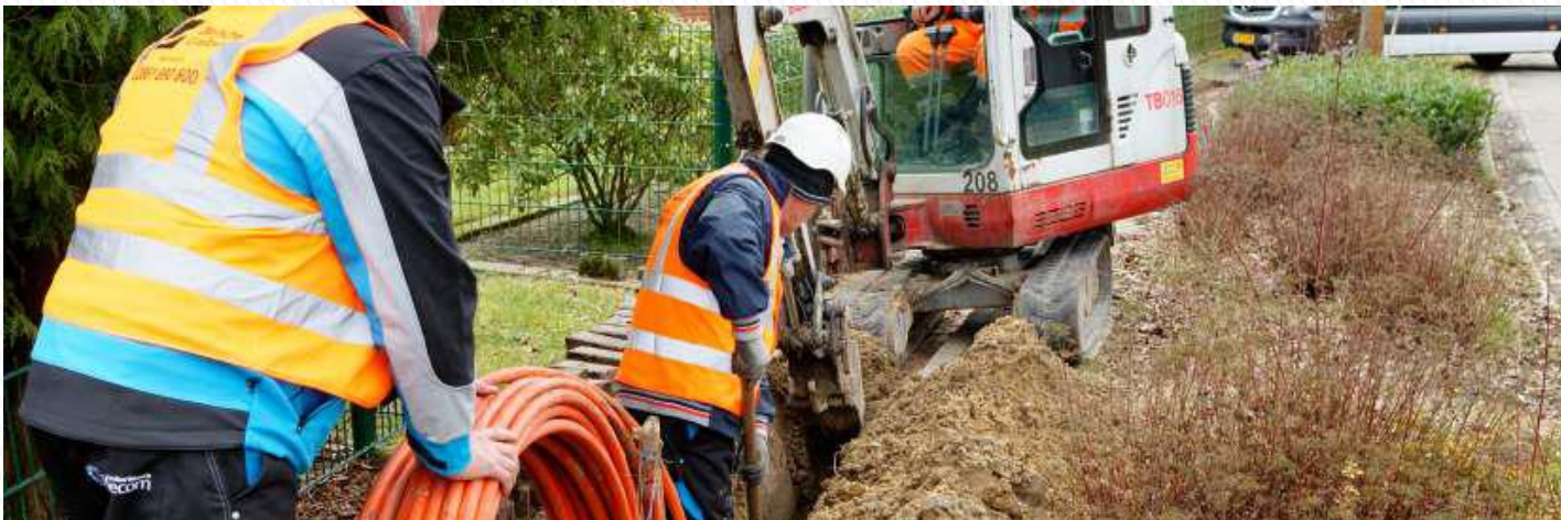
Figure – Protected microduct laid in open trenches
