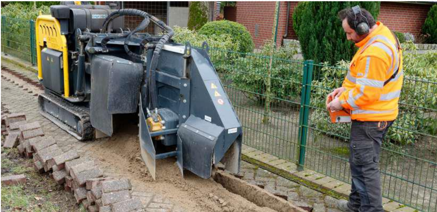
Figure - Micro trenching deployment technique
