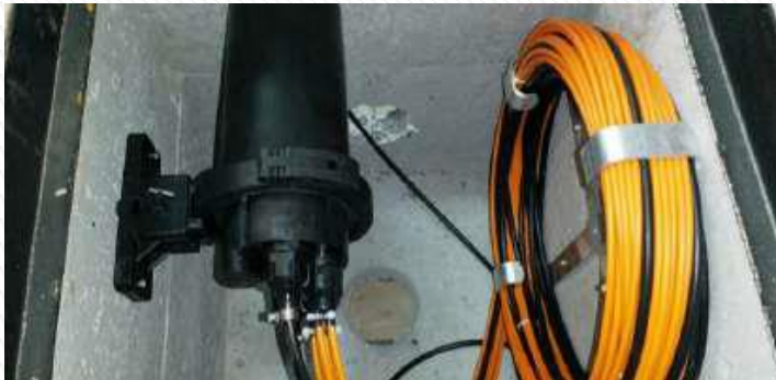
Figure – Splice closure and slack storage
